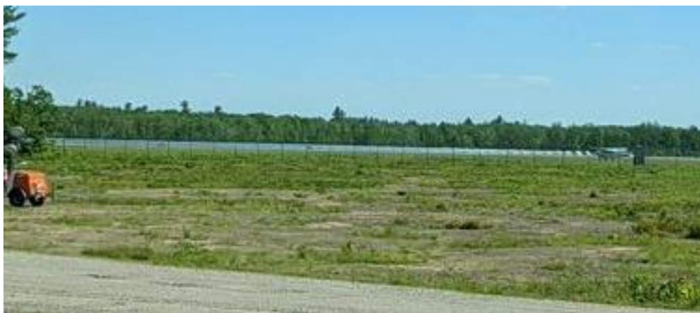
Figure 14 Sanford Airport Solar Farm
